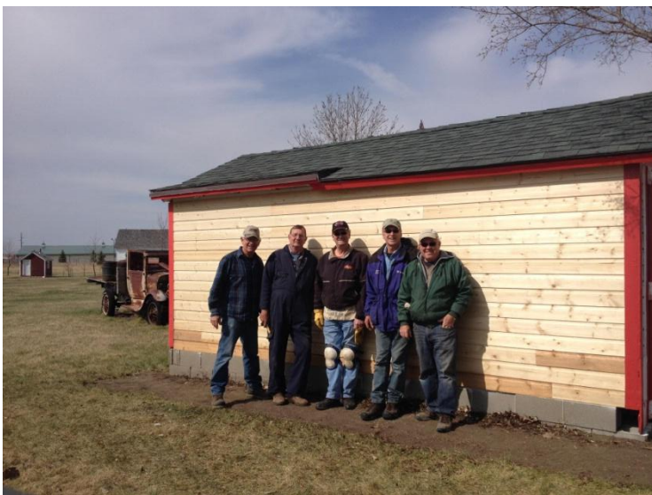
PAC crew replaces siding on storage shed at Buckstop Junction.
